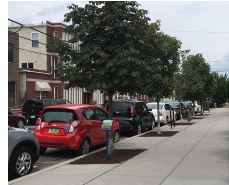
Stormwater Tree Trench
