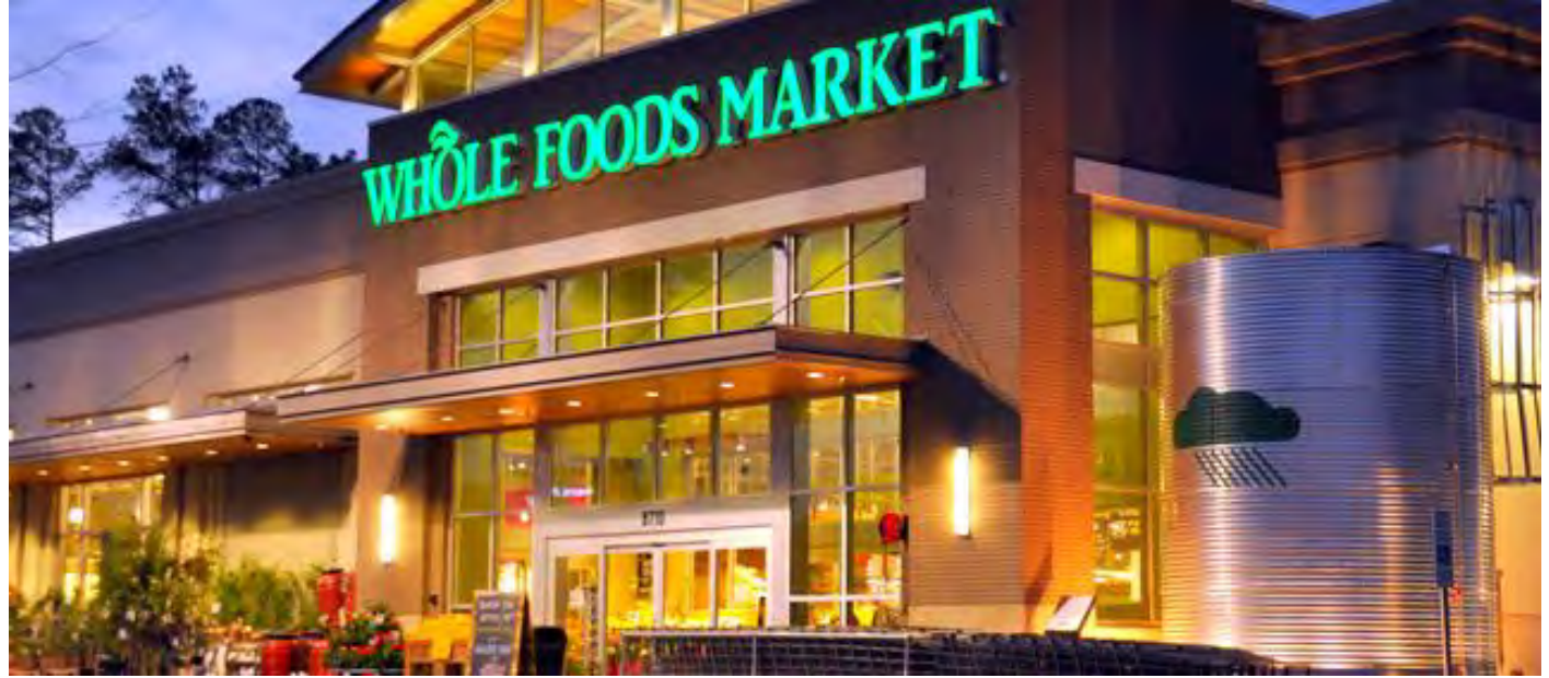
A 57,000-square-foot commercial development with an 800,000-gallon rainwater catchment system, including placement of a visible cistern.
