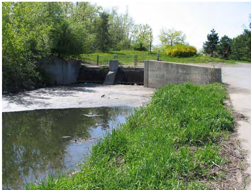
Figure B-3: Inlet to Underground Diversion of Scajaquada Creek Around Hoyt Lake
