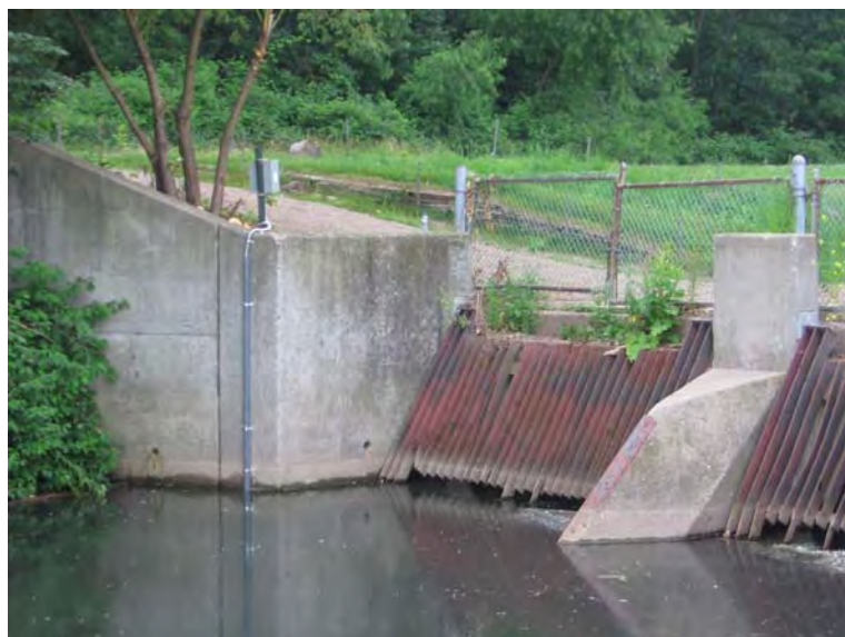
Upstream level sensor installation (stilling well and download box on concrete wall left of tunnel grates
