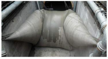
Figure 4 - Rubber Dam Example
