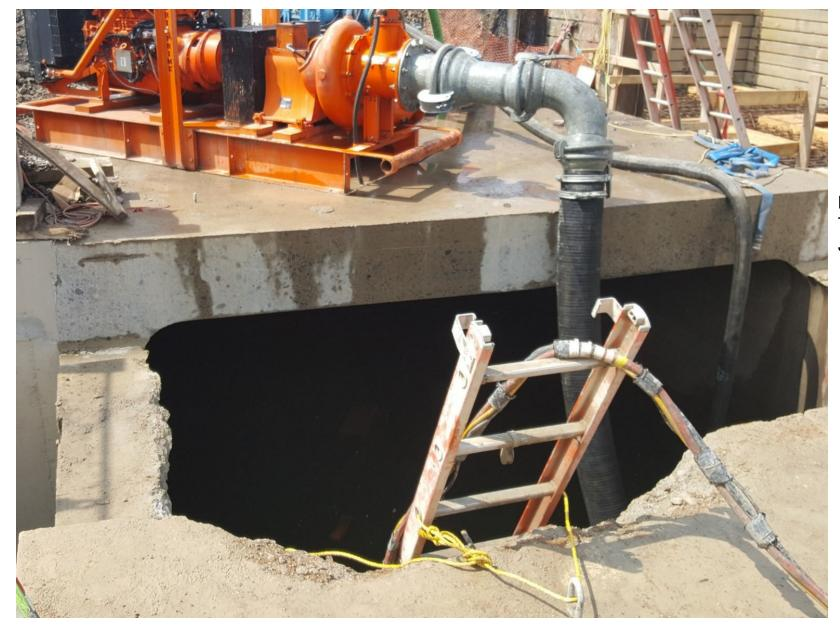
Dewatering Upstream of Temporary Bulkhead Weir June 2017
