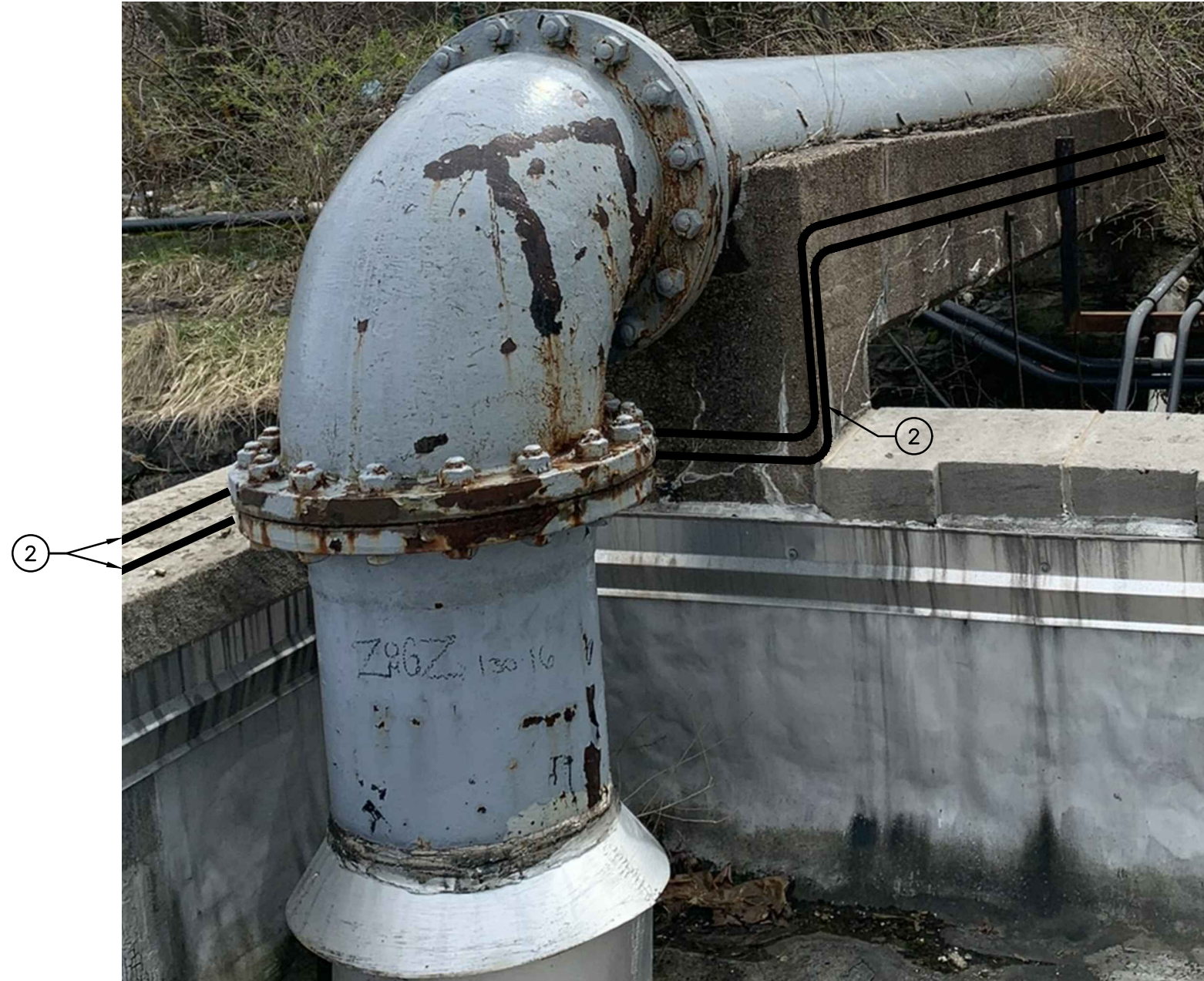
SECTION 2/E13 – CONDUIT ROUTING QUARRY PUMP STATION ROOFTOP AT EL 84.00 SCALE: NO SCALE
