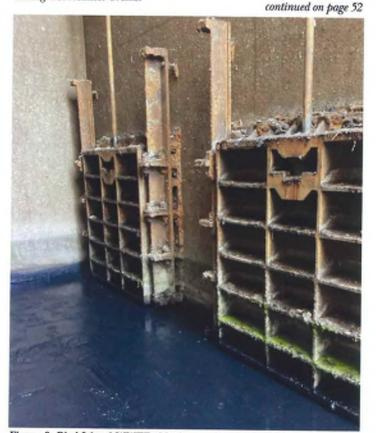
Figure 8. Bird Island WWTF chlorine contact tank sluice gates prior to removal. AECOM
