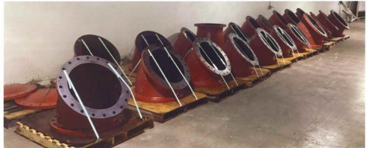
Figure 11. Bird Island WWTF large diameter ductile iron pipe fittings staged for installation.
