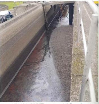
Figure 6. Bird Island WWTF aeration tank influent channel with accumulated grit and debris. AECOM
