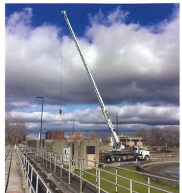
Figure 9. Bird Island WWTF chlorine contact tank sluice gates during removal. AECOM
