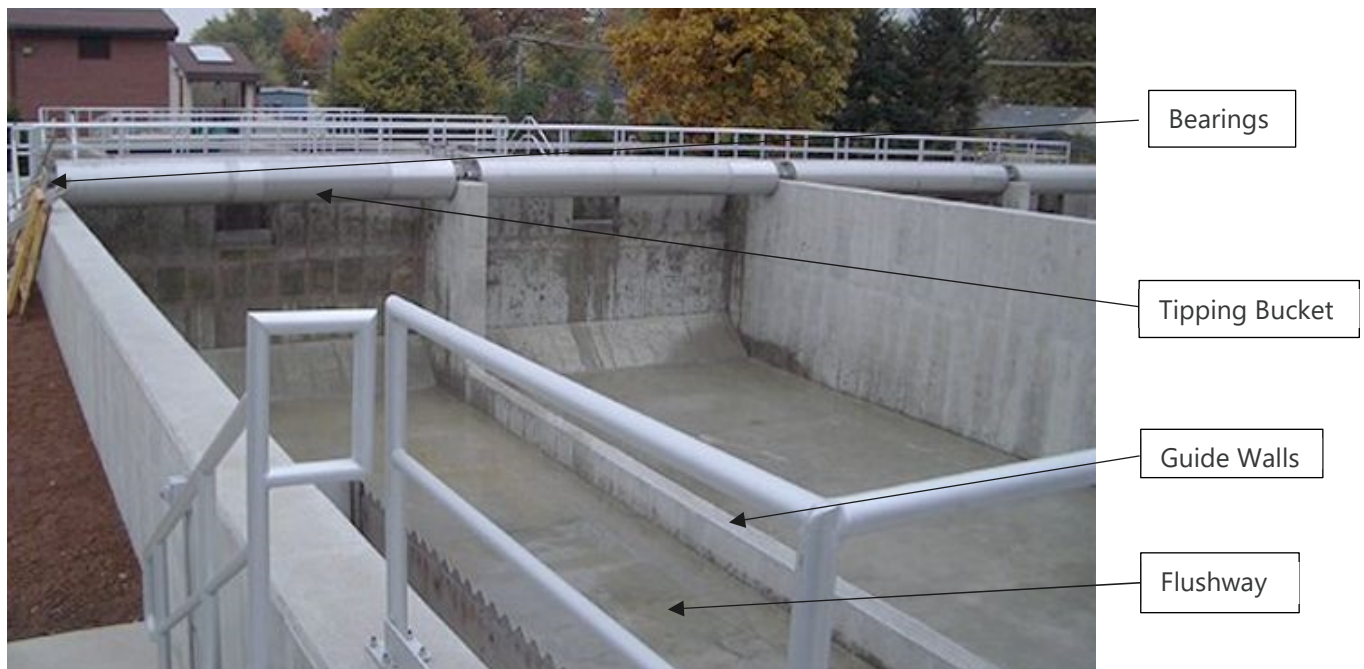
Figure 2-1: Tipping Buckets (source: Grande Water Management Systems)
