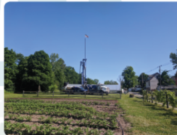
Wilson Streets Urban Farm well installation 2021
